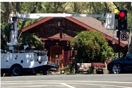
Safety camera installation at Highland and Moraga
